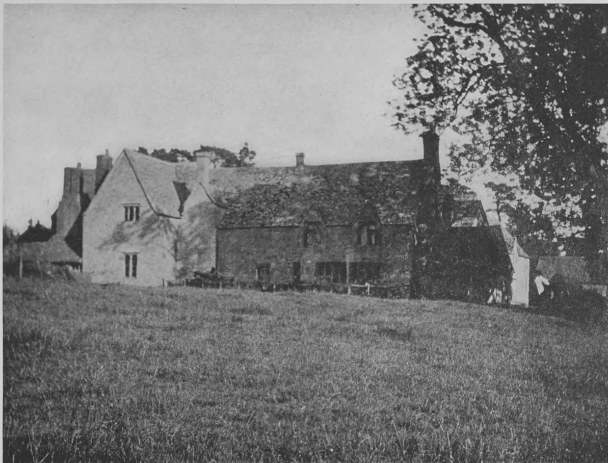
REAR OF LITTLE WOLFORD MANOR IN WARWICKSHIRE
